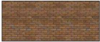
Body-brick in weston red multi by ibstock. stretcher bond with bucket-handle pointing in o.b.m.
